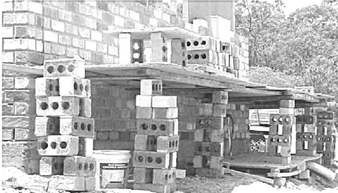
Concrete blocks as scaffolding
