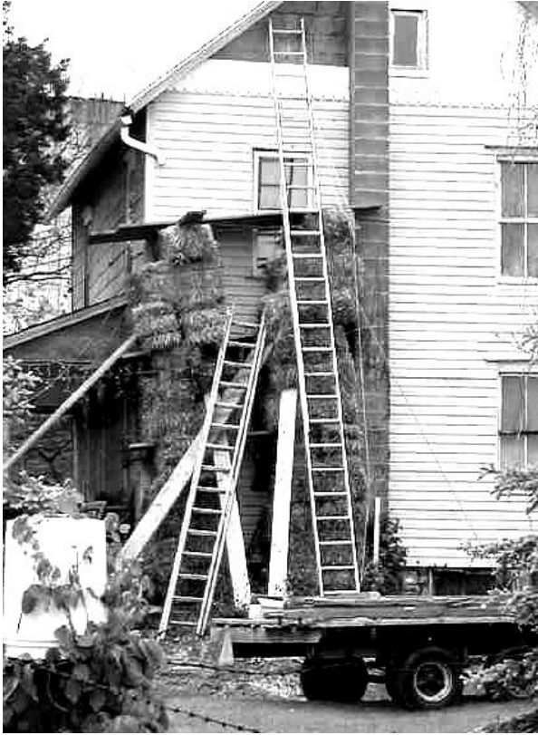
Hay bale scaffolding
