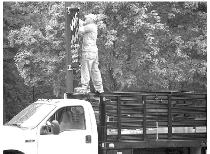
Truck rails as scaffolding
