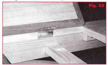
Remove the waste with a sharp chisel and screw the hinges in place (**Fig. 52**).
