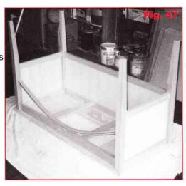
With the desk still upside down, insert the push rail through the slot in the front rail and through the slot in the location block.
